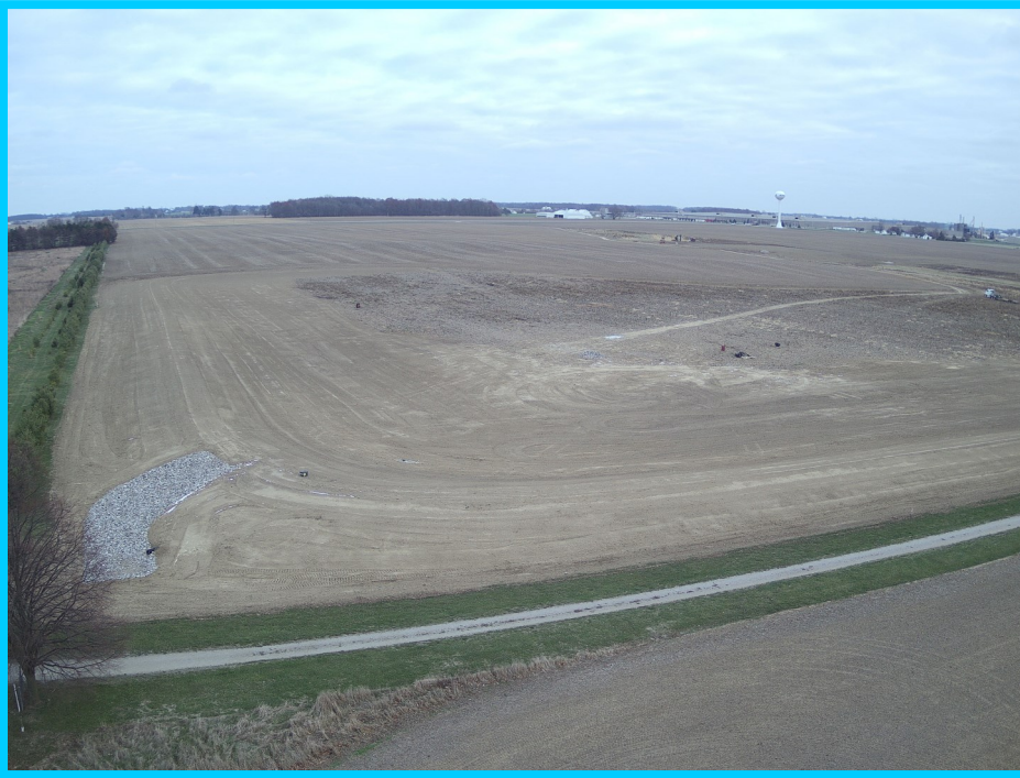
Southeast-facing view of newly constructed wetland pond. Outlet control structure and emergency spillway in left foreground.
